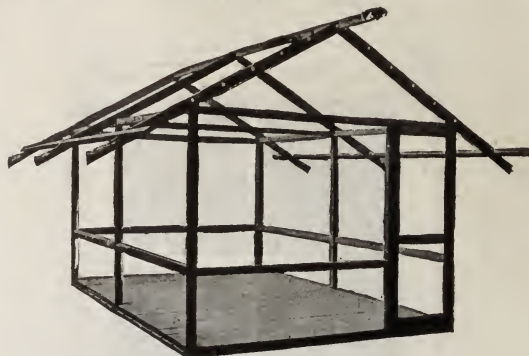
The above cut shows detail construction of the frame of the KHAKI WICKI-UP.
